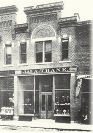
Trane Storefront La Crosse, Wisconsin 1891
